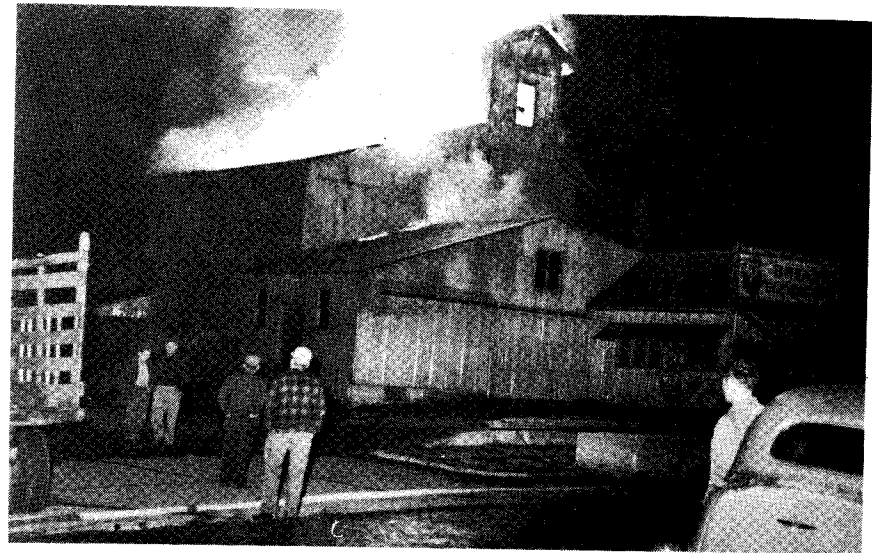
Bryant Elevator Co. was taken by fire during night in 1952. Living near the elevator, George Garlinger, standing by curb; Leo Ketchum, on sidewalk with hands in hip pockets; and John Hoskins, Mgr. were the first to arrive and hastily remove the important business papers from the office.
